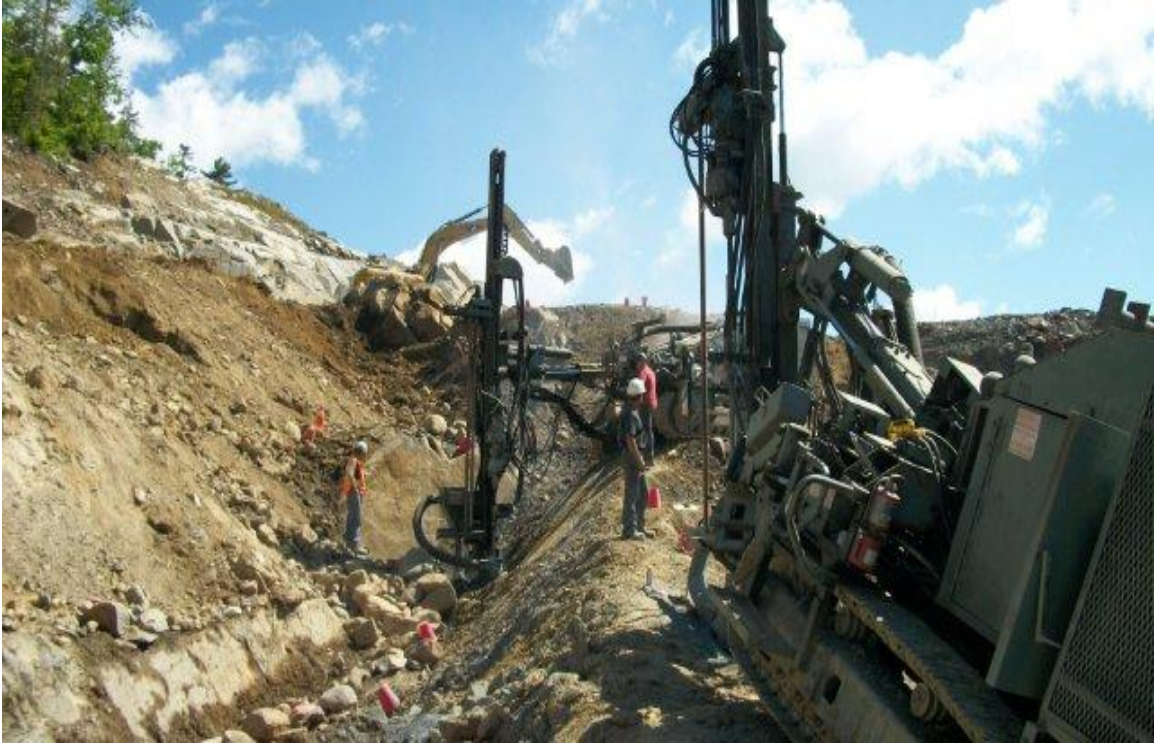
Blast hole drilling operations at the Shakespeare west deposit, May 2010.
